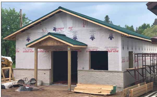
Louis A. Koenig Research Center in progress.
